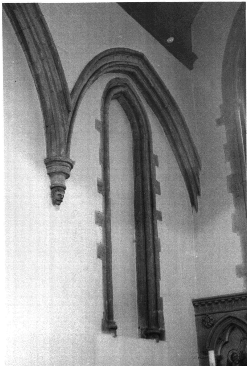
Sittingbourne. North wall of chancel.
